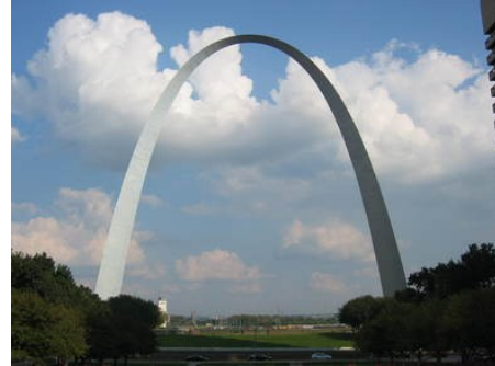
Fig. 3: The Gateway Arch is a flattened catenary.
